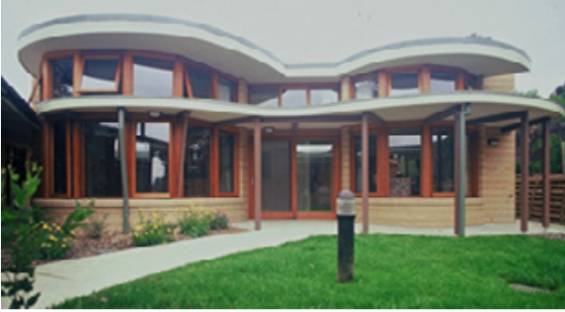
Path to lounge and dining area from bedroom areas.
