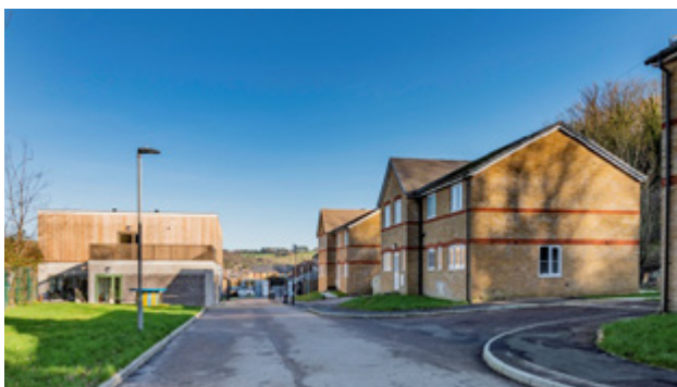
The people living with dementia are in houses on a residential street, and are free to move around the site using technology to alert staff to any issues.
