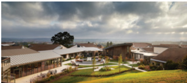
Accessible 'village green' courtyard with accessible routes from dining and activities room. Planters have been designed so that gardening can be conducted from a wheelchair and a number of 'memory nodes' have been included near to resting spots including a refurbished village water pump.
