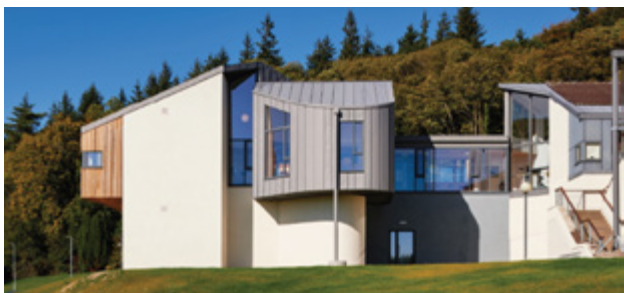
Although the facilities house over one hundred residents, care has been taken to ensure the architecture always reads at a domestic scale and feels familiar and homely.
